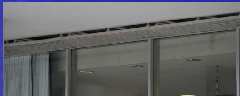
Installation of louvres above main foyer. Louvre blades are from 6mm thick aluminium flat bar welded to a recessed framework.
