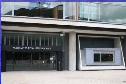
Installation of louvres adjacent stage entrance. Louvre blades are from 6mm thick mild steel flat bar welded to a recessed framework.
