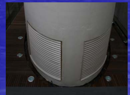
Installation of curved aluminium louvres. Design based upon our standard extruded aluminium louver
