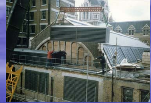
Acoustic Louvre Penthouse being craned into position – Natural History Museum
