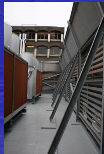
Structural Steelwork Supports
