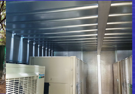
Acoustic Enclosure (ultra) designed for multiple air cooled condensers and heat pumps c/w high performance low resistance inlet and discharge attenuators & AP75 Acoustic Panels
