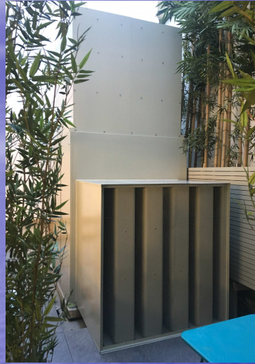
Acoustic Enclosure designed for vertical discharge air cooled condensers and heat pumps c/w high performance low resistance inlet and discharge attenuators & AP50 Acoustic Panels
