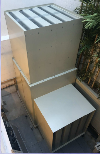
Acoustic Enclosure designed for vertical discharge air cooled condensers and heat pumps c/w high performance low resistance inlet and discharge attenuators & AP50 Acoustic Panels
