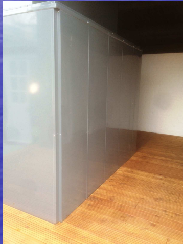
Acoustic Enclosure designed for multiple vertical discharge air cooled condensers c/w mid-range performance inlet acoustic louvres & mid-range performance discharge attenuators & AP50 Acoustic Panels
