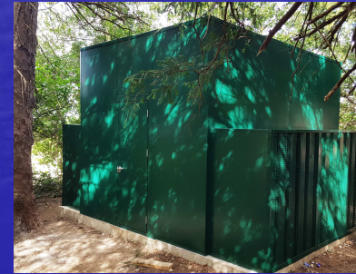
Acoustic Enclosure (ultra) designed for multiple air cooled condensers and heat pumps c/w high performance low resistance inlet and discharge attenuators & AP75 Acoustic Panels
