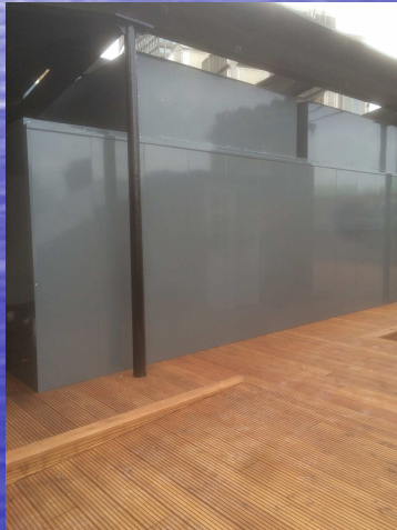
Acoustic Enclosure designed for multiple vertical discharge air cooled condensers c/w mid-range performance inlet acoustic louvres & mid-range performance discharge attenuators & AP50 Acoustic Panels
