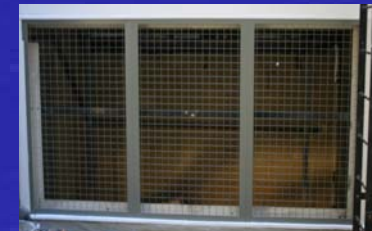
Specialist welded steel grilles and Waterloo WLS75/140 profiled aluminium louvres
